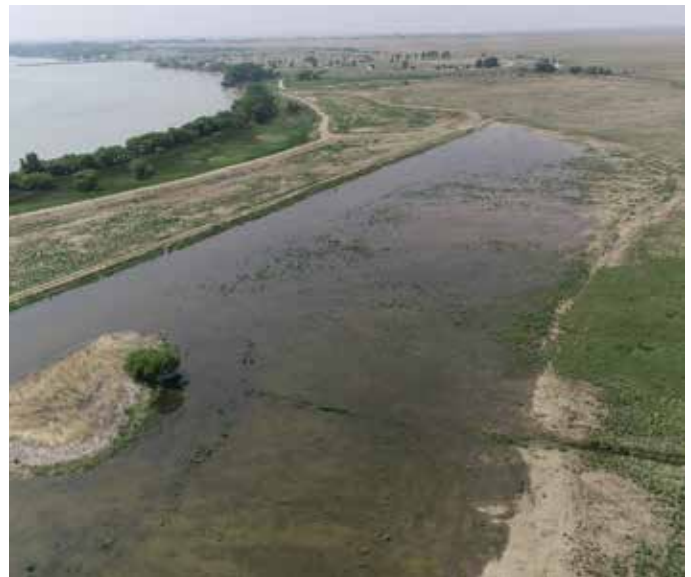
Wetland cells at Jackson Lake State Park after being filled for the first time. ©CPW
