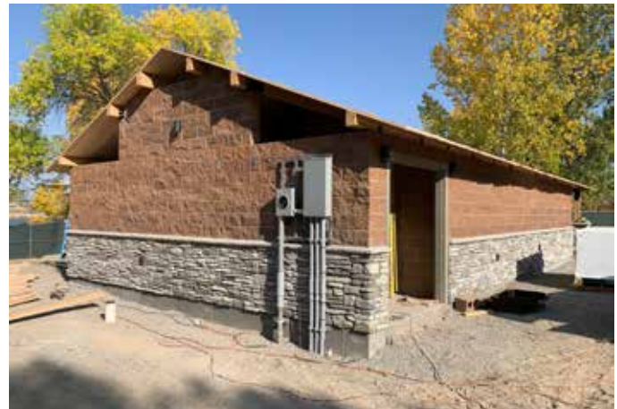
Highline Beach Restroom ©CPW
